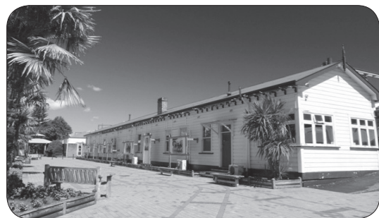
Te Kuiti Railway Buildings
